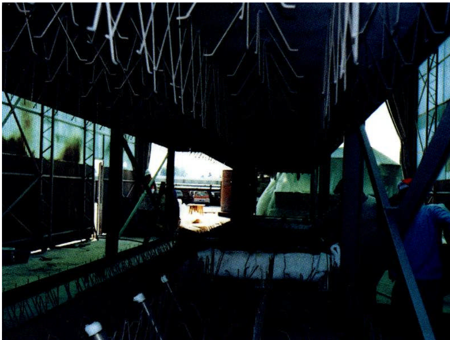
Stainless steel anchor system for insulating concrete lining
